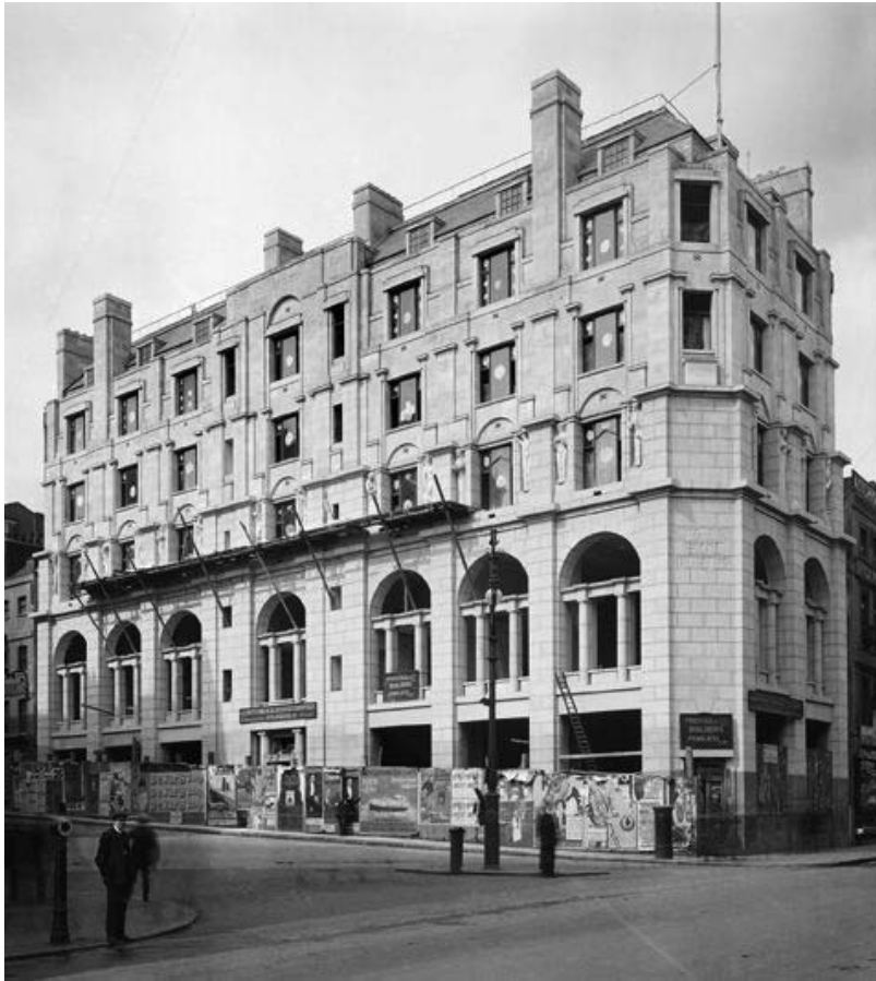
Fig. 6. The British Medical Association Headquarters (429 Strand, Westminster), designed by Charles Holden as partner of Adams, Holden & Pearson, 1908–9. Grey Cornish granite and Portland stone cladding a steel frame, slate roof. (Photograph courtesy of the British Monuments Record)
